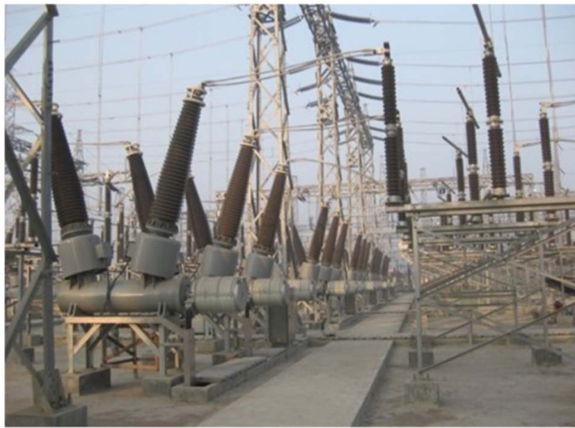
Fabrication of 230kV Gas Circuit Breaker(Jan.30, 2013)
