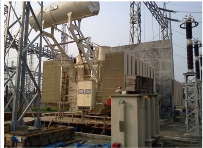
Fabrication of 230kV Transformer(Nov.09, 2012)
